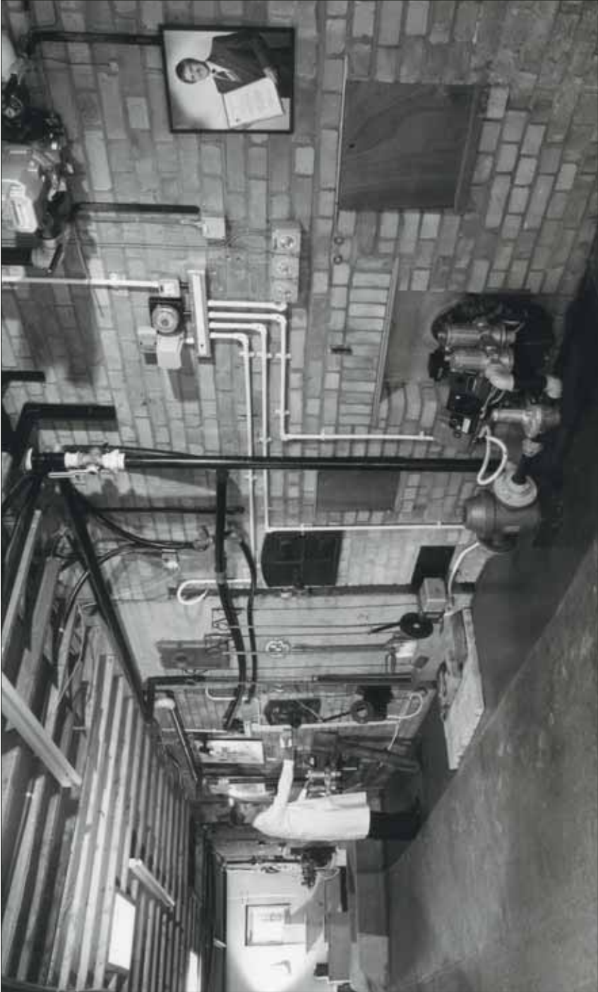
Clive Osborne in the stokehold, now transformed by modern technology. Compare this with the cover photograph of the same location.
